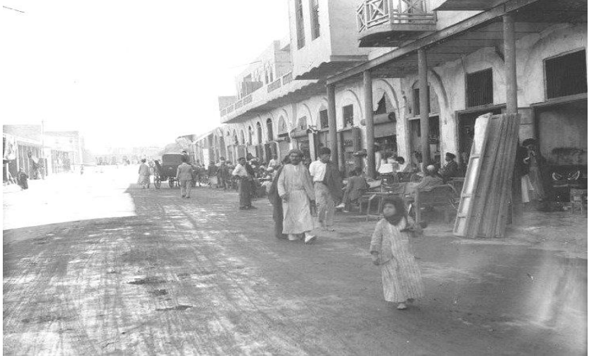
Figure (24) Iraq Kirkuk paving a street by the IPC in the late 1940s the black oil resulting from the liquidation of crude oil to spray the ground.
